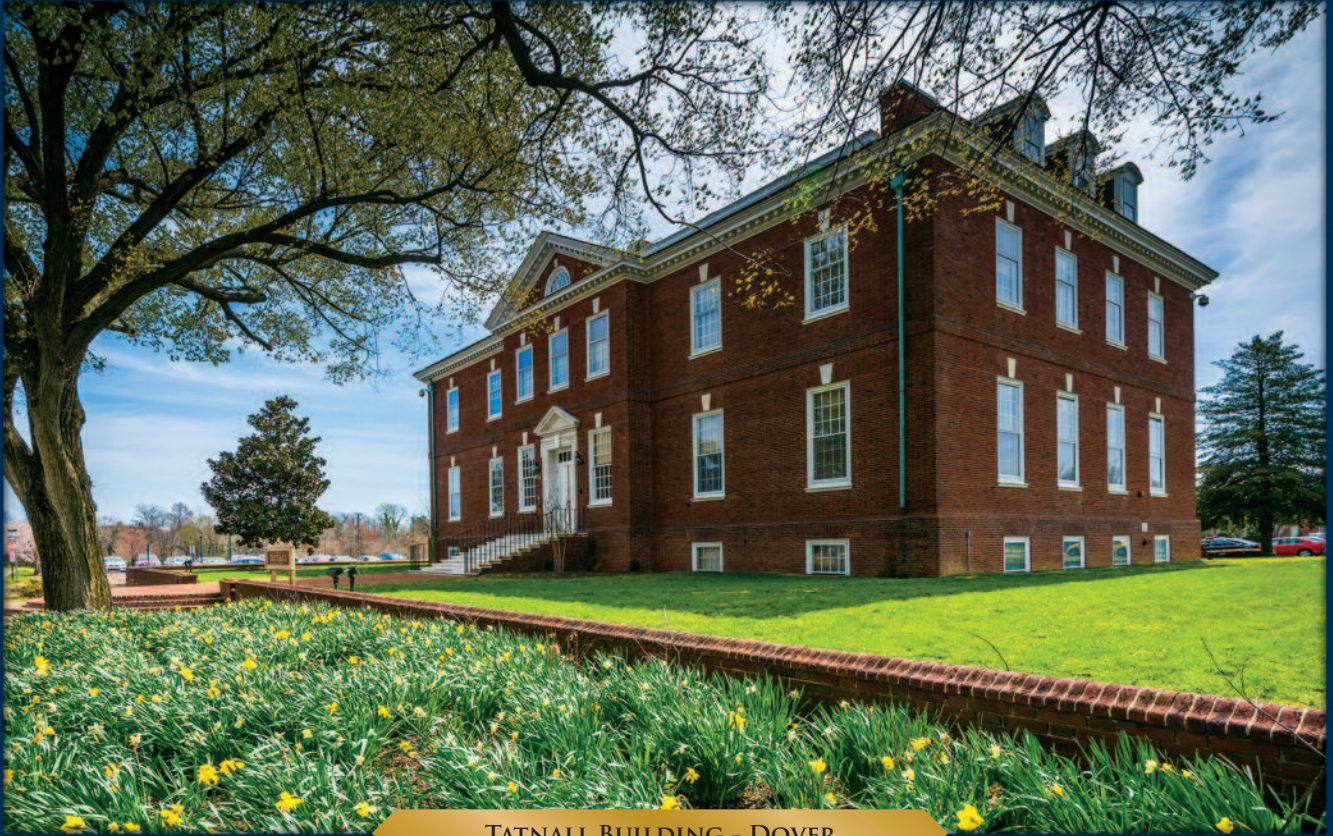
TATNALL BUILDING - DOVER
